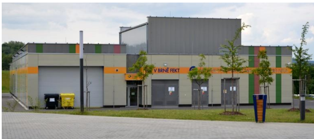
Fig. 6: External view of the CVVOZE PowerLab
